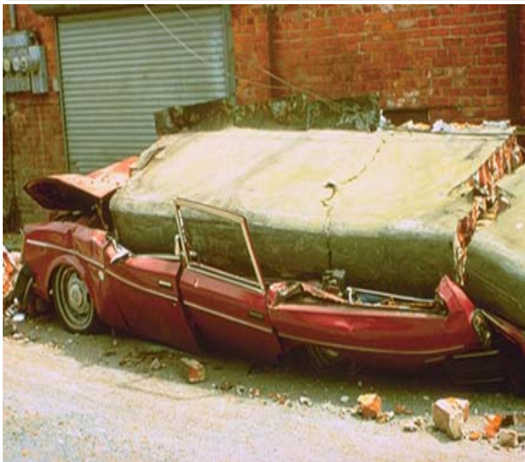
Damage Caused by Unreinforced Masonry (URM) Building FEMA PHOTO
