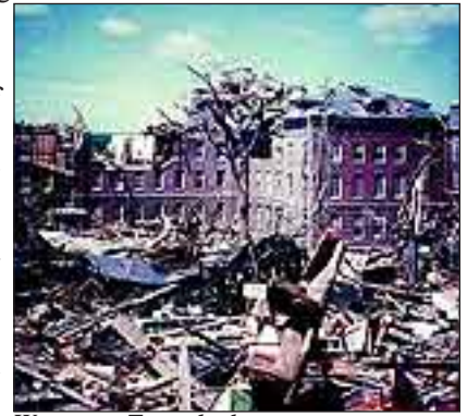
Worcester Tornado damage IMAGE: NOAA
