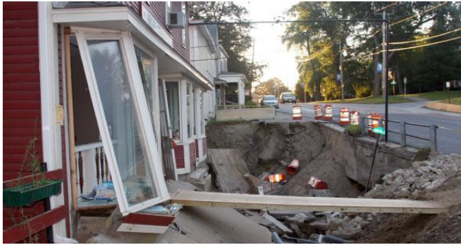
Building facades destroyed by floodwaters following Tropical Storm Irene FEMA PHOTO
