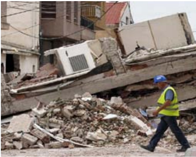
A rescue worker walks past rubble from collapsed buildings in the center of Lorca, Spain. BBC PHOTO
